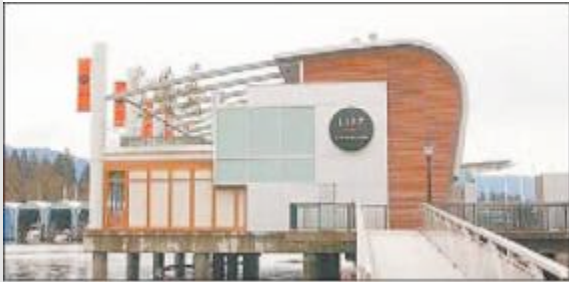
Horizontal-banded rare tropical woods contrast with corporate aluminum panels at the Lift Restaurant at Coal Harbour..
