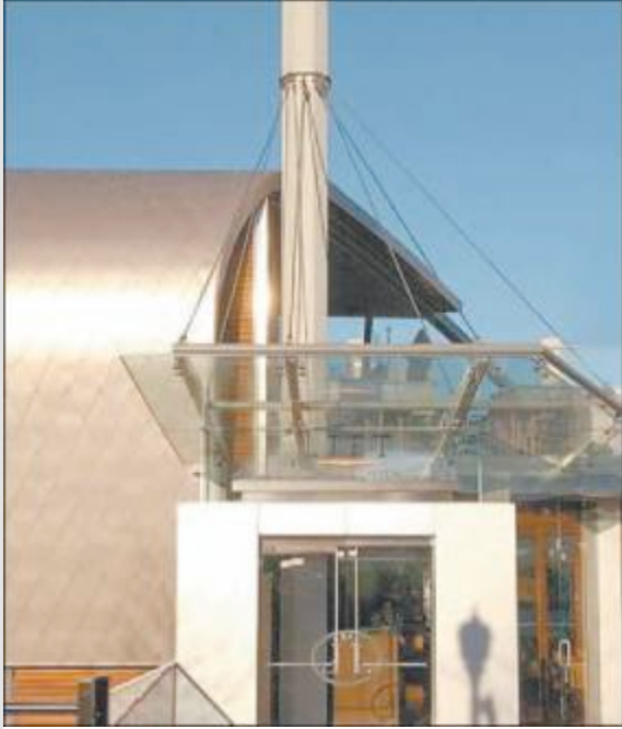
Matte-finished metal panels and a fir ceiling frame the downstairs fast food operation's outdoor cafe at Kits Beach's Watermark. Cables hold up the glass canopy at the yacht-inspired Lift's front door. The building features a curving roof, raised exterior deck.
